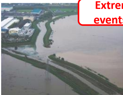
Flood damage “Hirota river, Aichi” (provided by MLIT)
